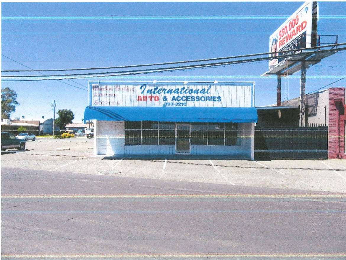
WEST ELEVATION – Front of Building from Across Street
