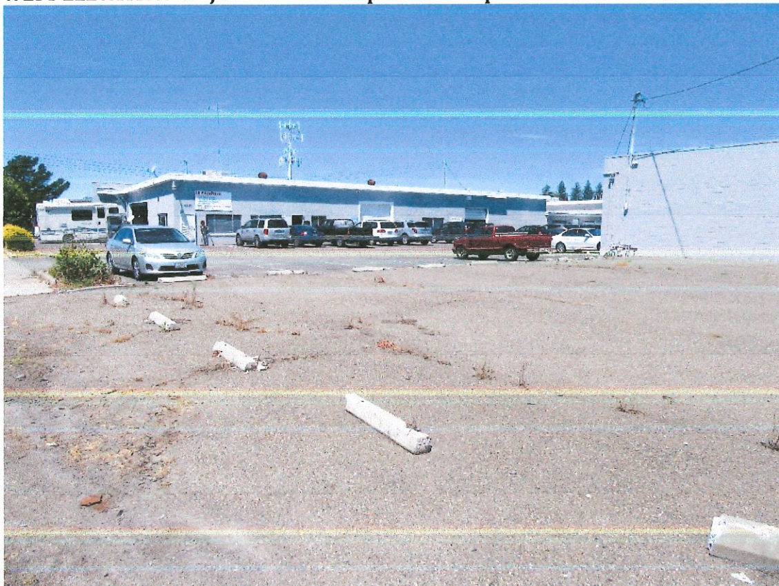
WEST VIEW – From Far Side of Street
