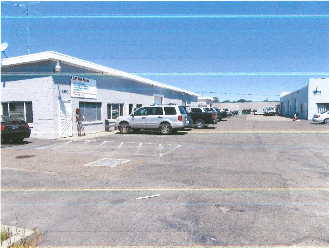
NORTH WEST VIEW – South Half of Front of Building
