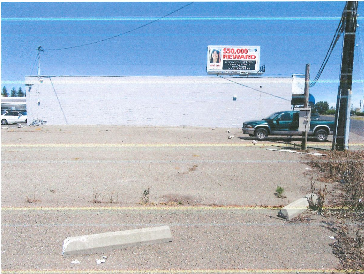
NORTH ELEVATION - Adjacent Property to the South
