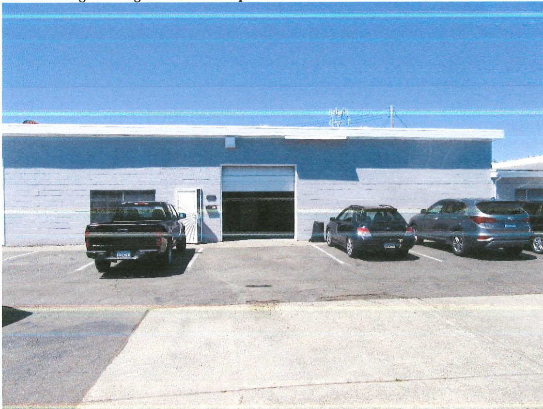
WEST ELEVATION –Adjacent Tenant Improvement Space
